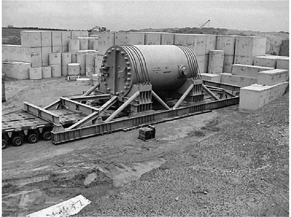
Figure 4: Delivery of a Large Reactor Vessel to the LLRW Trench at the Barnwell Disposal Facility
